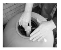
6. Using filter sand or Zeo-Clor, carefully place the sand into the filter tank. Ensure that the sand is slowly poured into the tank until the laterals are completely covered. Continue placing the remainder of the sand into the filter tank making sure as you go that the plastic disc is keeping the centre stem in the centre of the filter tank opening.
