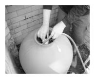
9. The multiport valve may now be attached to the sand filter tank.
